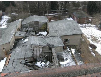
Figure 10: Building planned for demolish.
