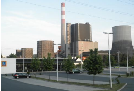
Figure 5: Shut down power plant in the Region Voitsberg.
